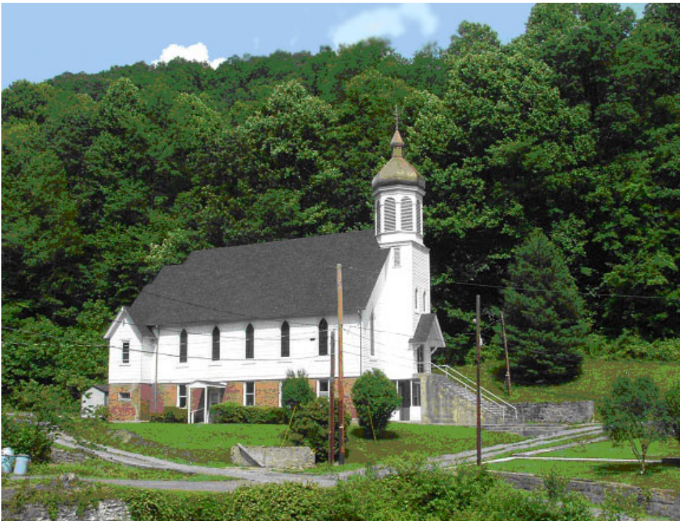
Local land mark – Prior St. Mary's Orthodox Church, Elkhorn, West Virginia, established in 1912.
